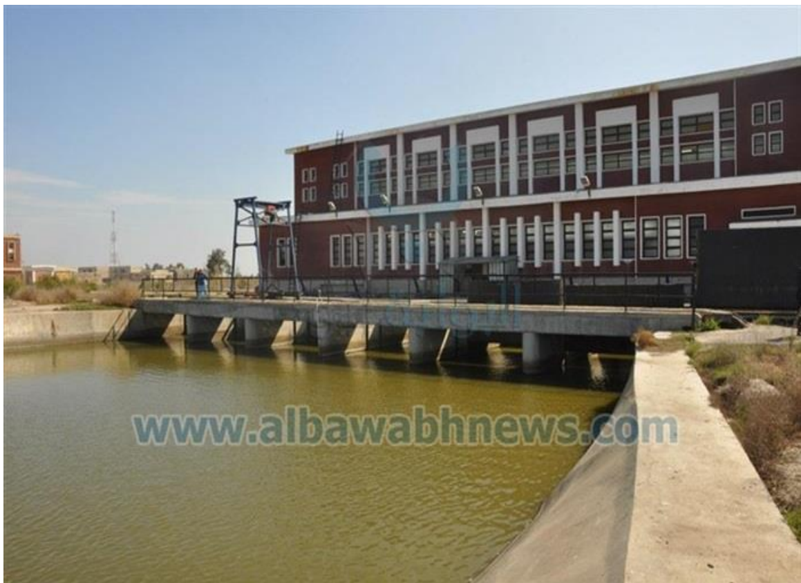
Pump station no. 7
